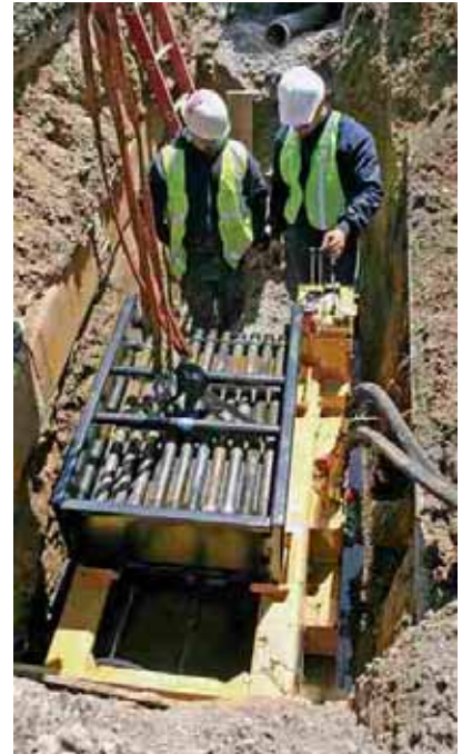
A hydraulic rod bursting unit. Picture courtesy of Earth Tool Inc/U Mole Ltd.
