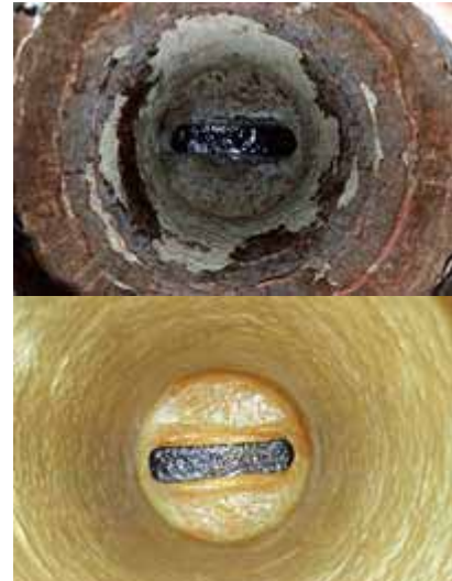
CIPP manhole rehabilitation before (top) and after (bottom).
