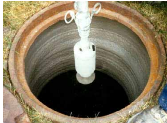
Spray lining of a manhole with a specially designed spray nozzle.
