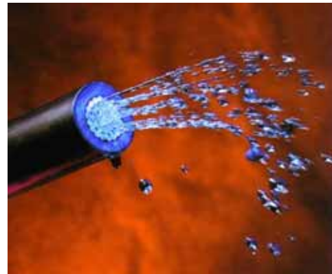
Silicone inject applied to impregnate a water damaged cable.
