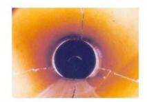
Figure 2: Host pipe condition II [DWA-A 143-2].
