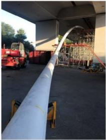
Fig.14: PE pipe, pulling phase
